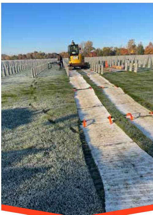
Deployed Trax provide access while protecting the ground conditions.
