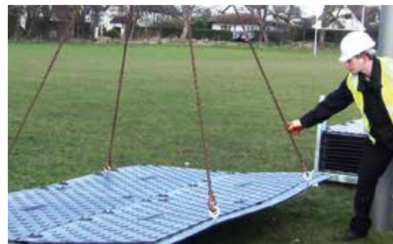
For faster installation mats can be joined in fours and lifted into place
