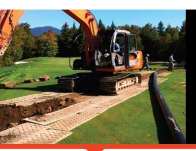
Designed for equipment, AlturnaMATS have an aggressive tread pattern to maximize grip, prevent ruts and create stable pathways. Available in 3 different tread patterns: cleats on both sides for maximum traction and grip, smooth on one side to simplify storage use on hard services and smooth on both sides to protect flooring on inside jobs or as a landing for a flat blade to scoop up material.
