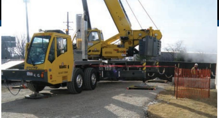
Nabholz Construction, Rogers, Ark., uses SafetyTech and FiberMax crane pads on top of improved ground that is firm, drained and graded.
